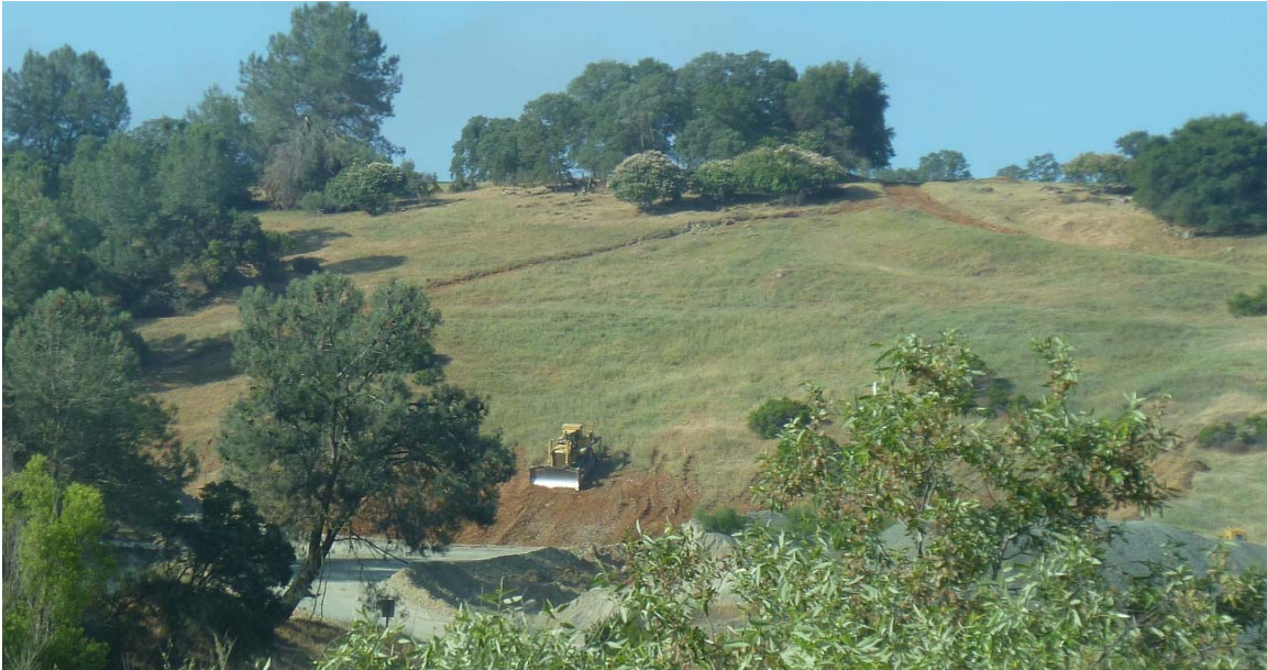
Site grading, May 2015
